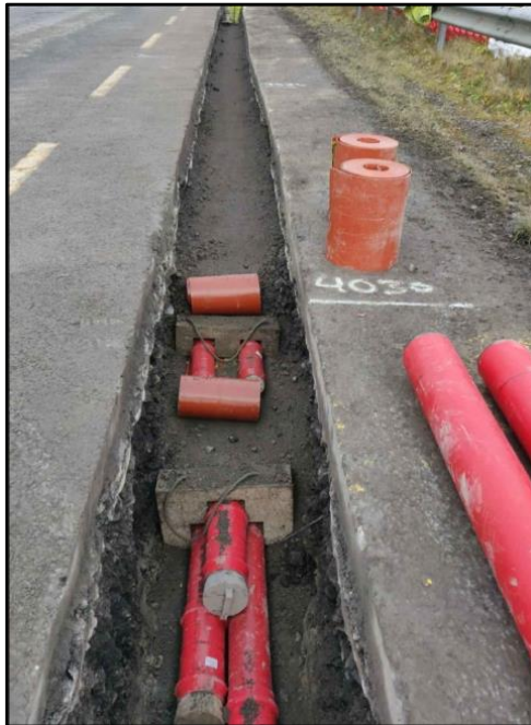
Plate 2-1 110Kv Cable Trench View
