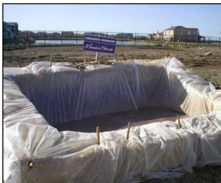
Plate 3-1 Typical concrete wash out areas
